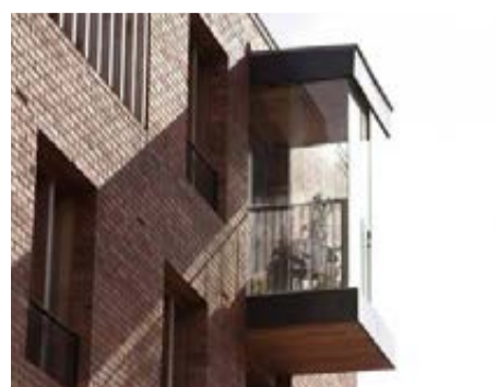
Articulation of the elevational line, Timberyard, Dublin
