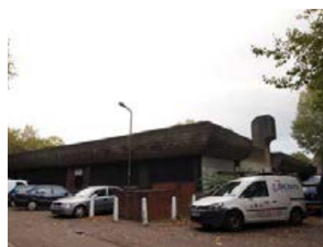
Existing energy centre
