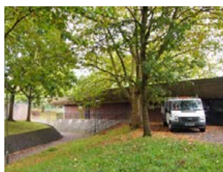
Existing energy centre
