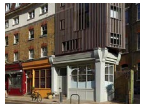
An active ground floor level, Alex Monroe Studios, Southwark
