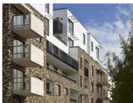
Expression of balconies and articulation of rooflines, Kilburn, London
