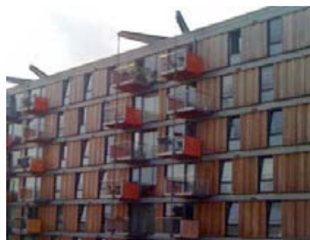
Prominent, lively frontage, Adelaide Wharf, Haggerston
