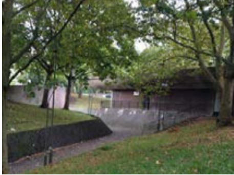
The existing sunken path leading to the energy centre
