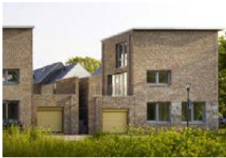
Off street bay parking at gable ends, Molenplien, Netherlands
