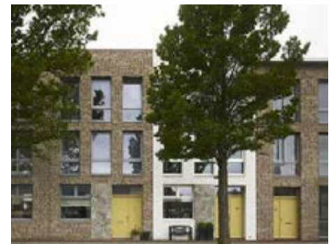
Main entrances to the street., Molenplien, Netherlands.
