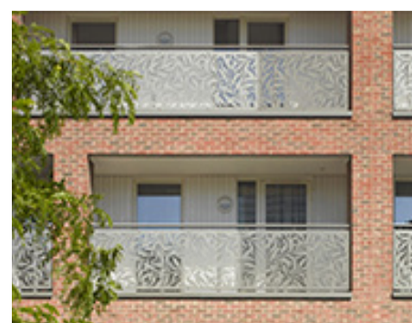
Inset balconies to mid level apartments, Canning Town
