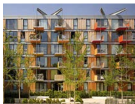
Prominent, lively frontage, Adelaide Wharf, Haggerston
