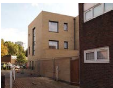
Existing material palette at phase 1B development
