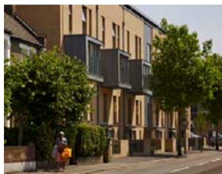
A mix of flats and maisonettes, Hammond Court, Waltham Forest, London
