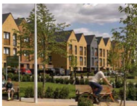
Animated facade, material use & roofline on main frontages, Kidbrooke Village, Phase 1
