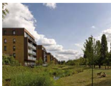
Overlooking the main green space with pronounced gables and frontage. Kidbrooke Village Phase 1
